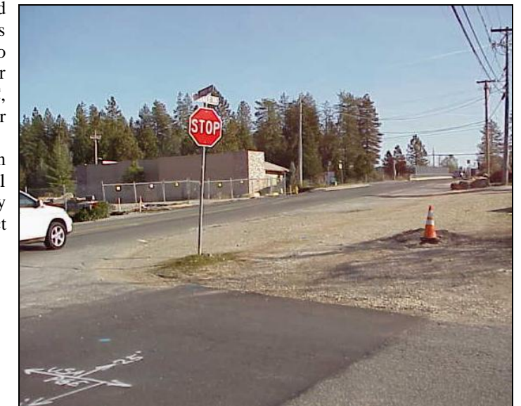
Utility relocation in progress for the Dorsey Drive Interchange project
