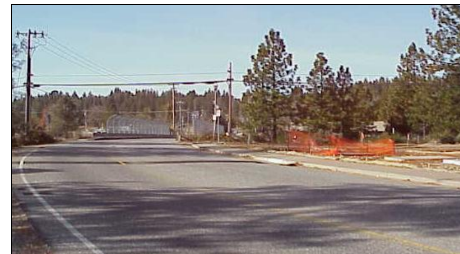
Preconstruction work near the Dorsey Drive overcrossing nearly completed
